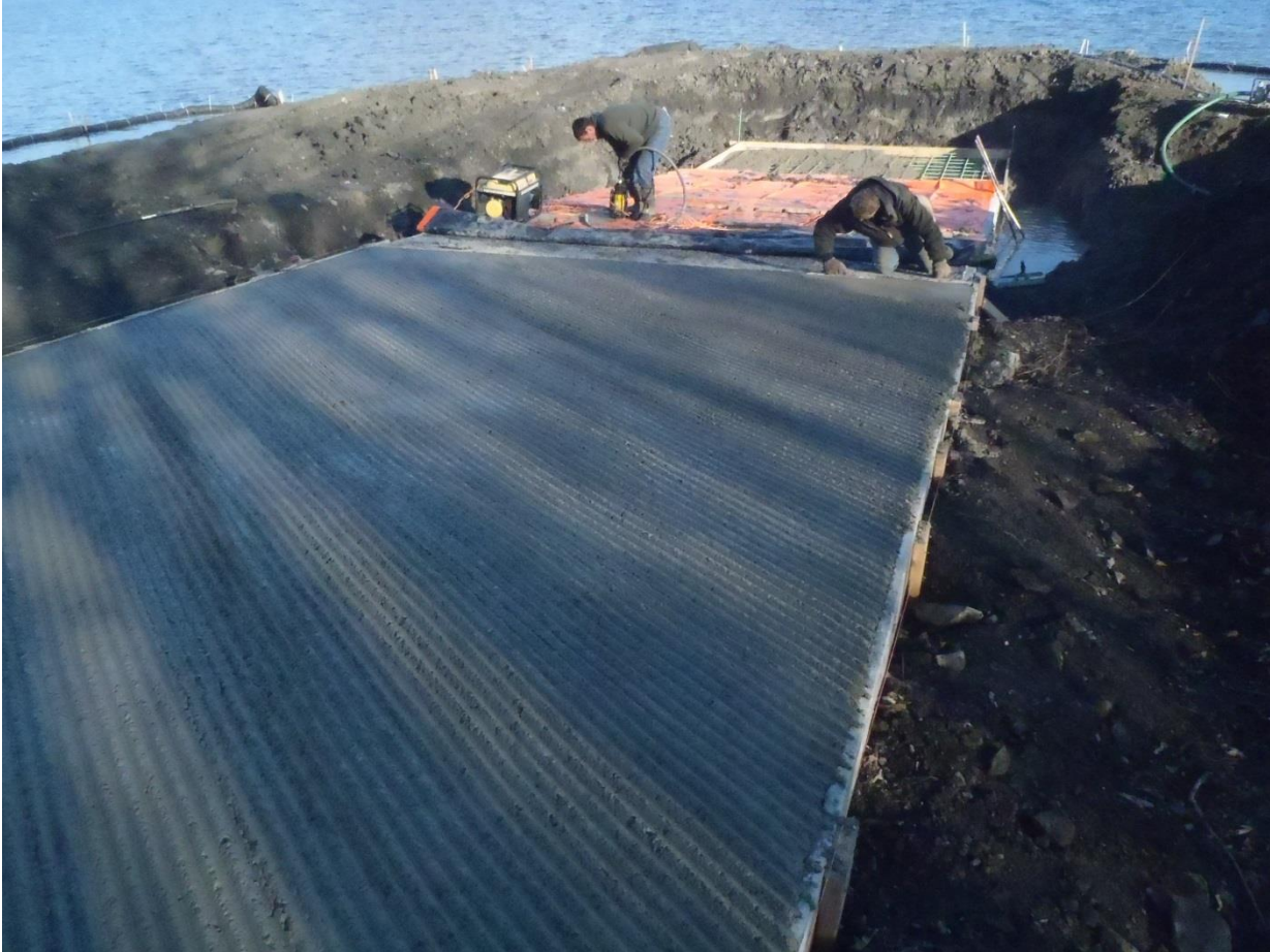
Figure 3. Pouring the concrete at the Dillenbeck Bay Fishing Access Area in Alburgh, VT. The ramp was formed and poured December 2016 and the project was completed April 2017. This popular fishing access area used to have a very shallow gravel ramp, which made launching at this site after early July difficult to impossible. Now anglers, boaters, and waterfowl hunters can utilize the ramp into the fall.
